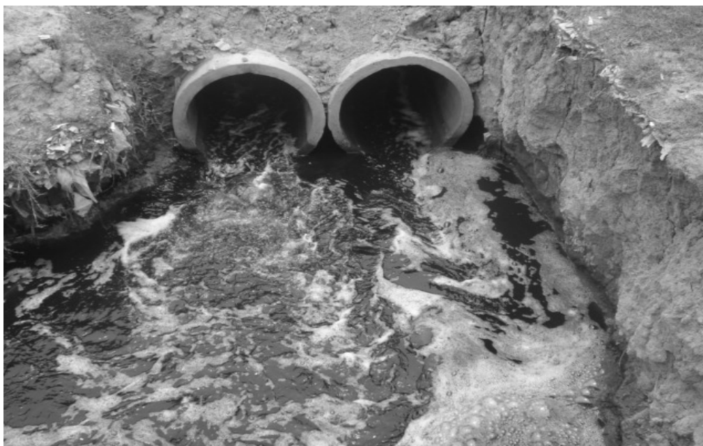
Fig. 1. Open discharge of industrial wastes in South Dhonua, Sreepur, Gazipur
