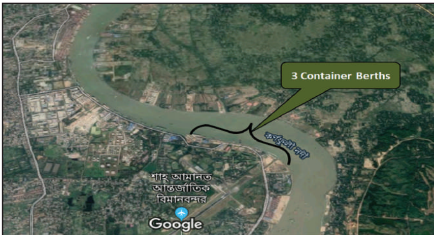
Figure 16: Patenga Container Terminal Site (Source: Google)
