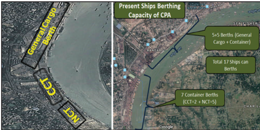
Figure 15: Number of Berths and Location (Source: Google Earth)
