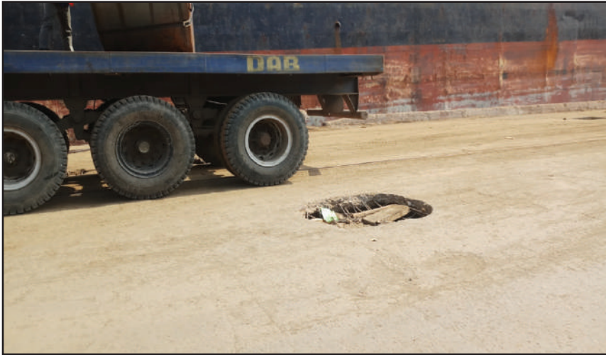
Figure 17: Present Condition of GCB Area (Source: Primary)
