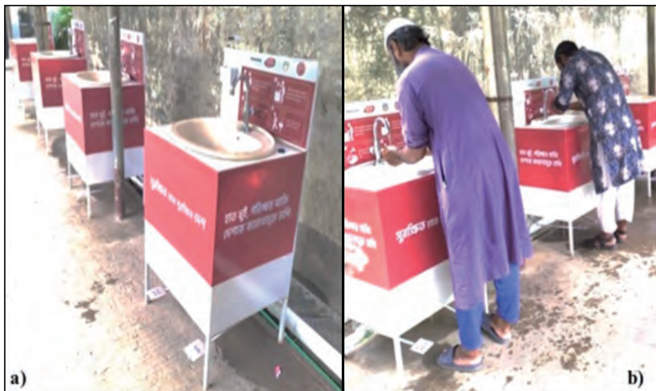
Figure:1. a) Newly installed pedal operated hand-washing basins at the entrance of National Institute of Nuclear Medicine & Allied Sciences. b) All patients and attendants wash hands before queuing up
