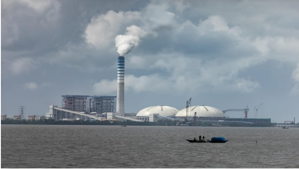
Figure 3.1: View of the Andharmanik river near the PTPP showing reduced fish activity due to pollution from the thermal power plant.
