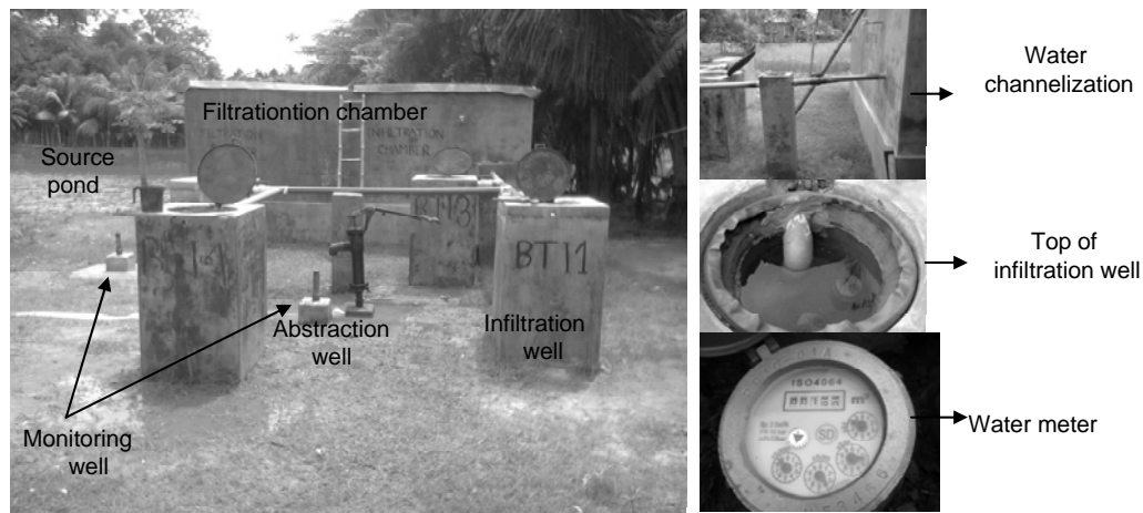
Fig. 1. A complete managed aquifer recharge scheme at Batiaghata, Khulna.
