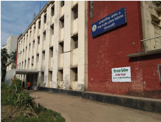
Figure 1: The Four-storied building in which COVID-19 laboratory is located.
