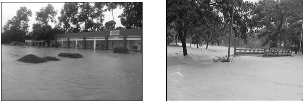
FIGURE 4: FLASH FLOOD AFFECTED SCHOOL (LEFT) and AFFECTED ROADS (RIGHT).
