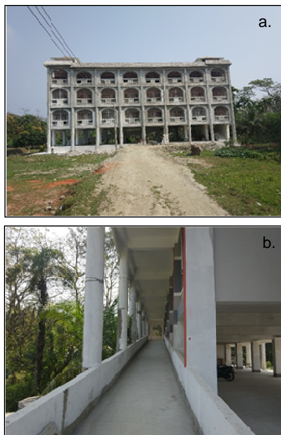
Photograph 1: The College to be Used as Cyclone Shelter: a. outside of the shelter b. ramp of the shelter.
