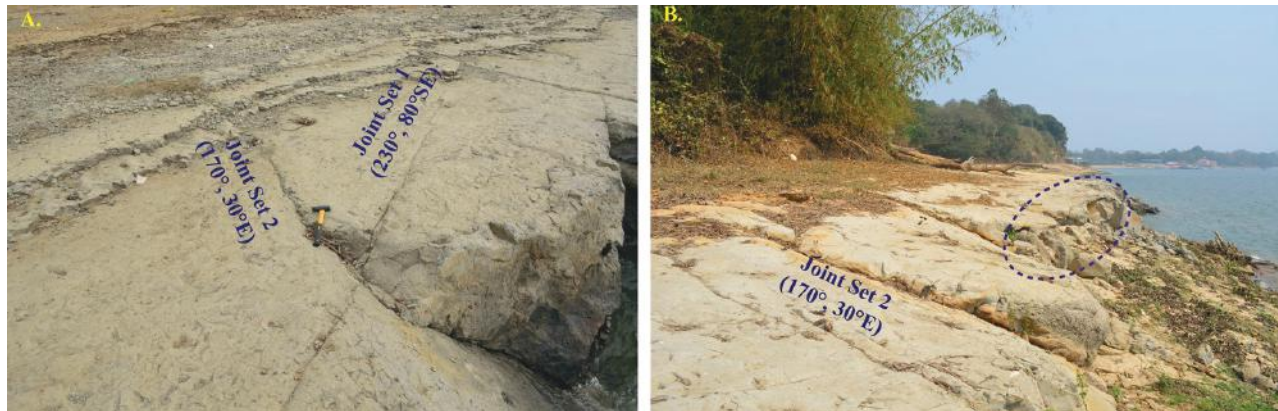
Figure 7: (A) Two Sets of Crisscross Joints and (B) The Blocks of Rocks Breaking Away (Inside Blue Ellipse) Along the Joint Planes
