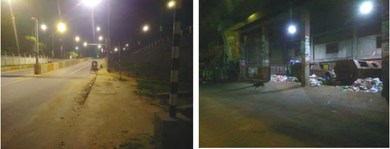
Figure 16: (Right) In Postogola, a Bridge Ramp was Constructed Over the WASA Network Node. (Left) In Jatra-bari a Garbage Storage Station was Constructed Supposedly Over the Chamber. The Road Sections were Surveyed and no Significant Signatures were Noticed. Our Conclusion is Derived from Eye Witness Accounts of Locals and WASA Personnel
