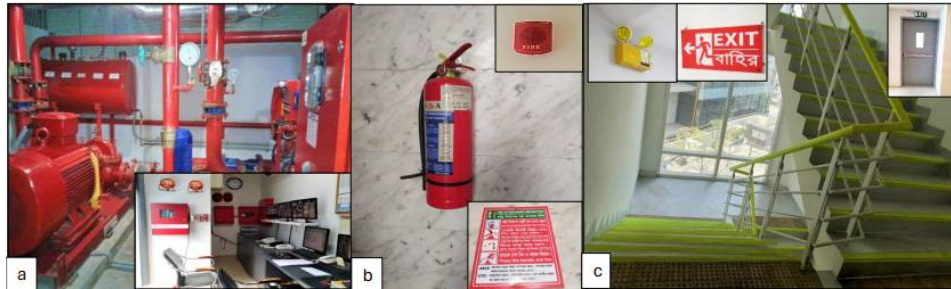
Fig. 3. Illustration of excellent to good examples of well-equipped control room (a. inset), hydrant with pressurize valve (a.); Fire extinguisher (b.), fire alarm (b. inset upper right) and direction of extinguisher user procedure (b inset lower right); Well-ventilated exit (c.), emergency light (c. inset upper left), exit sign (inset upper middle) and exit doors (c. inset upper right). (Source: Fieldwork, 2019-20)
