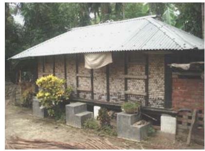
(g) Outside house storage structure (gable) made of bamboo, tin and wood
