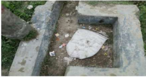
Figure 8. A bag with sand is used as a lid of outlet
