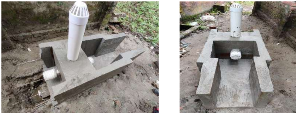
Figure 3. Final structure of modified buried pipe riser with attached air vent
