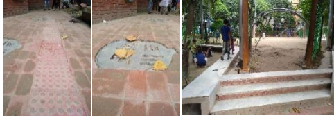
Figure-08a: Tactile indicator, Obstruction and steps at SIP
