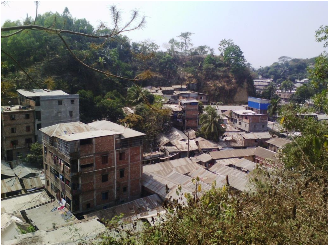
Fig 9: Showing the housing development happened on hill by hill cutting in Motojorna area.
