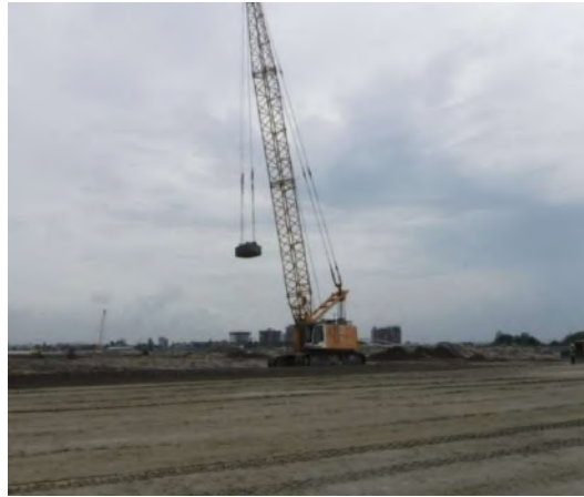
Figure 5: Execution of Dynamic Compaction Work
