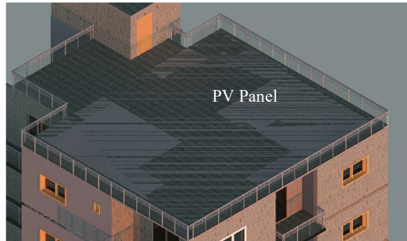
Figure 11: Provision of PV Panel at Upper Roof.
