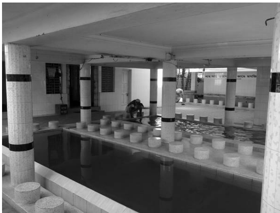
Fig. 5. Ozu facilities in Bandar Mosque.
