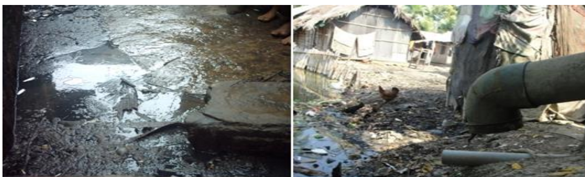
Fig. 6. Poor or no drainage system in the slum (Source: Field Survey, 2011)
