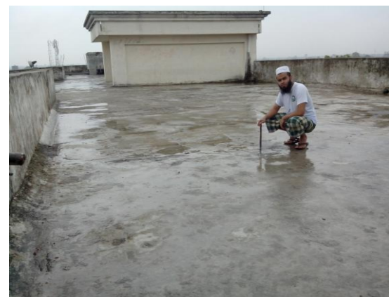
Fig. 5. Roof Catchment in modern building
