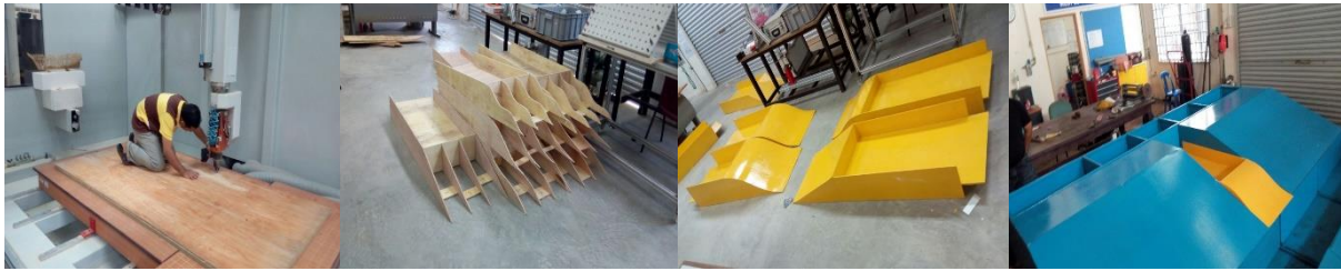
Fig. 4: Ramp shapes construction and assembly process
