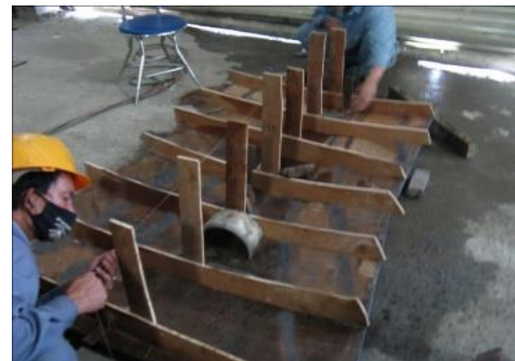
(e) Verify the longitudinal curvature of the K1 plate
