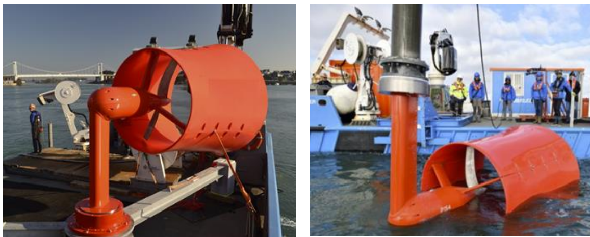
(a) Commissioning/ installation of the tidal turbine
