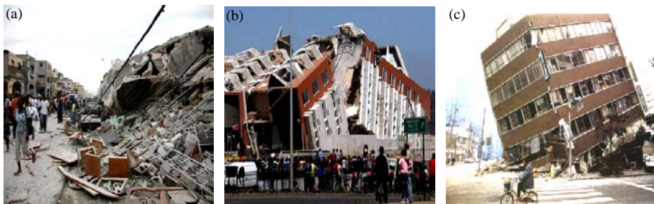
Fig. 18. Photographs showing the degree of building damages (a) Haiti, (b) Chili and (c) Kobe earthquakes.
