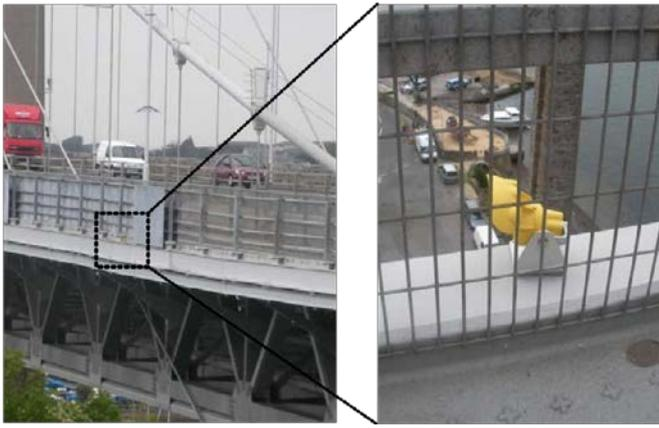
Figure 7: Reflector in bridge deck [25]
