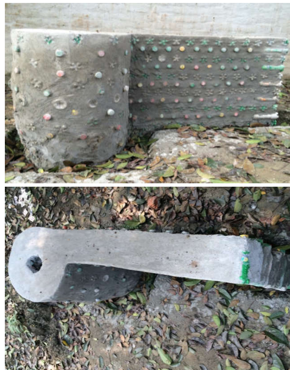
Figure 8. (i) A column and part of a wall constructed with plastic bottle bricks; (ii) View from the top of the column and the wall.
