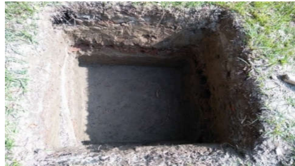
(a) Soil digging to 3 feet
