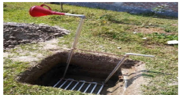
(b) Placement of aluminum tubing in soil
